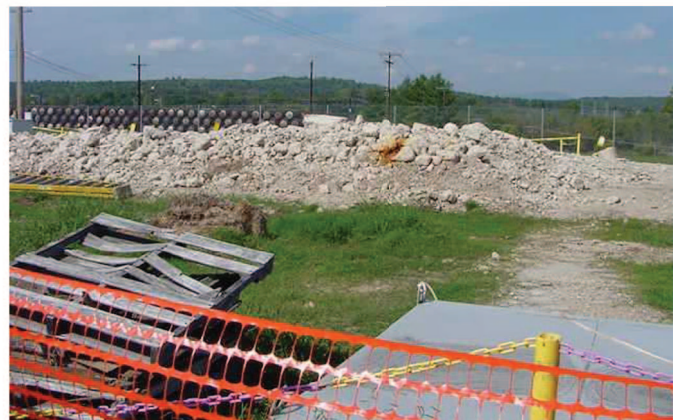
After D&D. Building rubble awaiting disposal.
