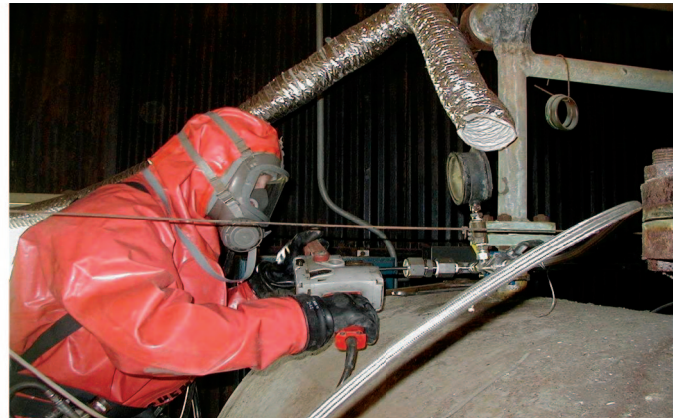
During D&D. Taking fluorine gas measurements prior to removal.
